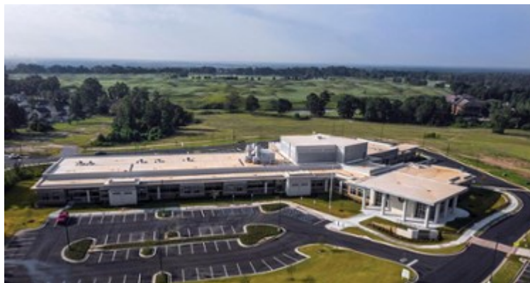
Aerial view of the ADPH-BCL building complex in Prattville, AL
